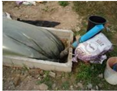
Photo 7: The inlet to the biodigester
