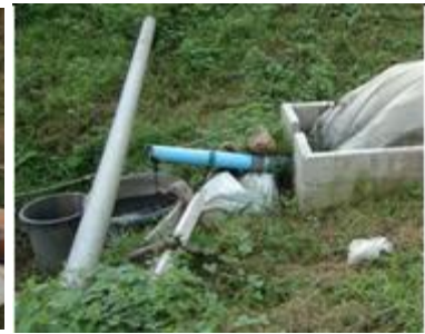
Photo 8: Collecting the effluent
