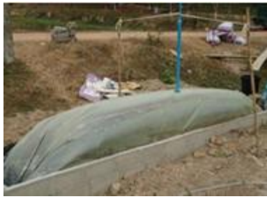
Photo 6: The tubular polyethylene biodigester
