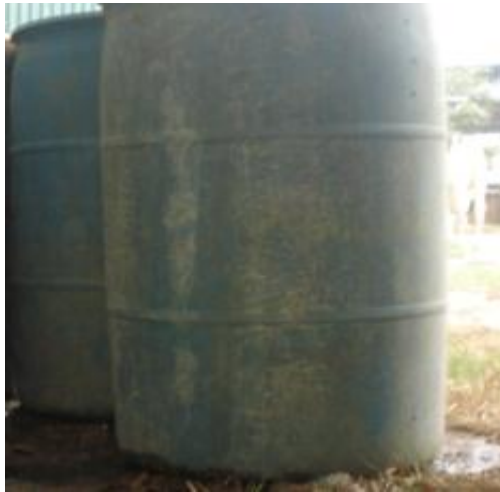
Photo 9: Effluent storage before applied
