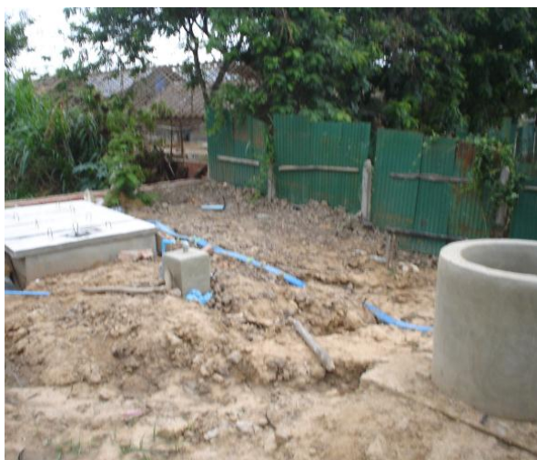
Photo 6: Concrete biodigester
