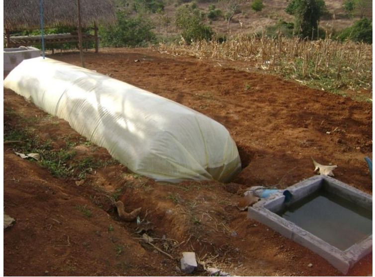
Photo 5: Effluent from the plug-flow tubular polyethylene biodigester
