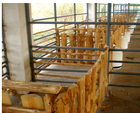
Photo 1. Pigs individual pens made from wood with concrete floor
